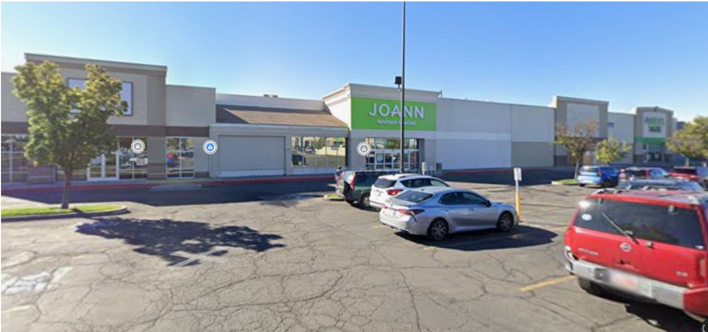
Figure 1, Parking lot view of 172 E University
