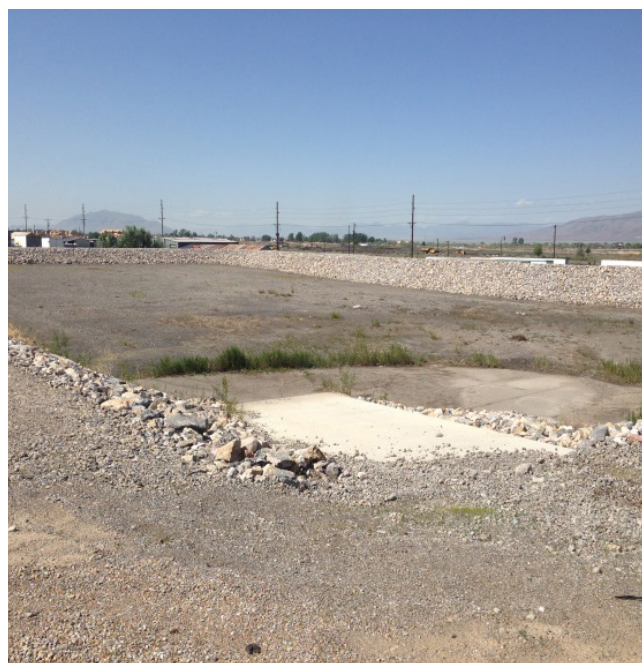
800 North Detention Pond
