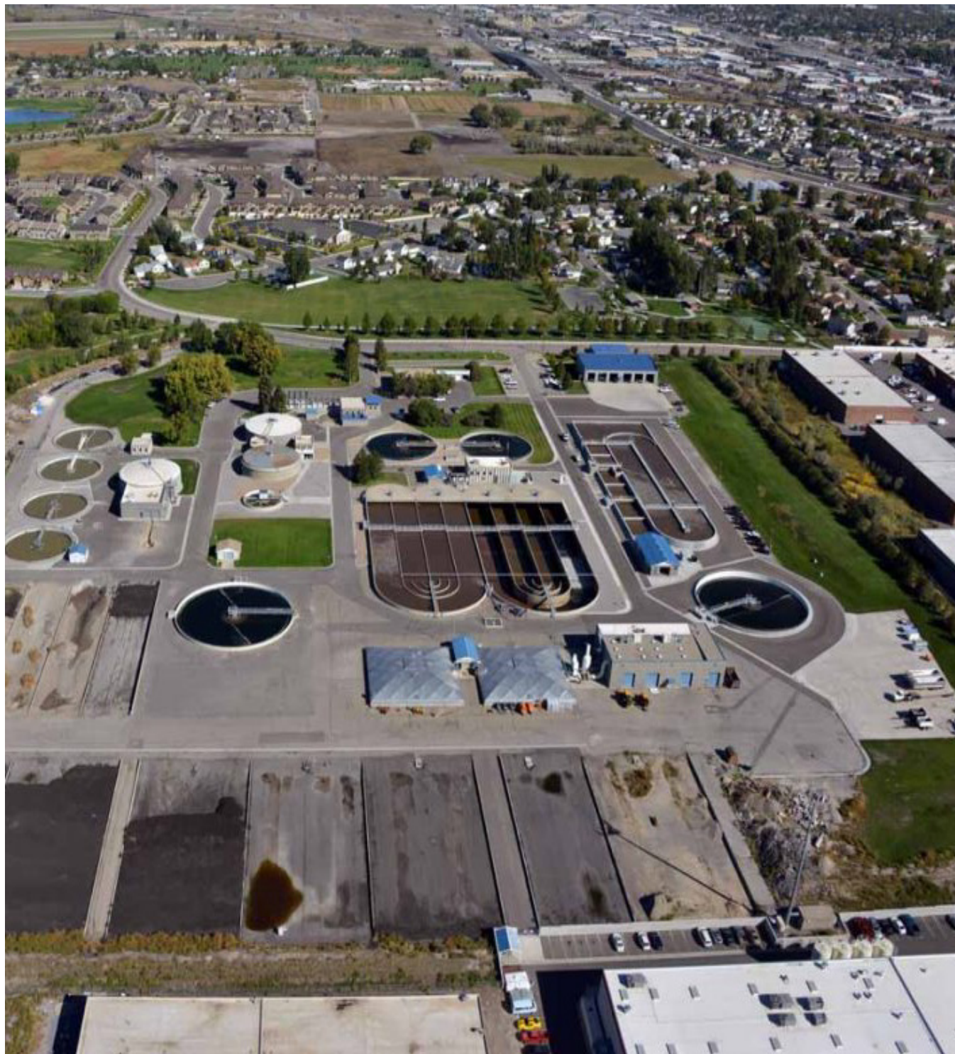
Water Reclamation Plant
