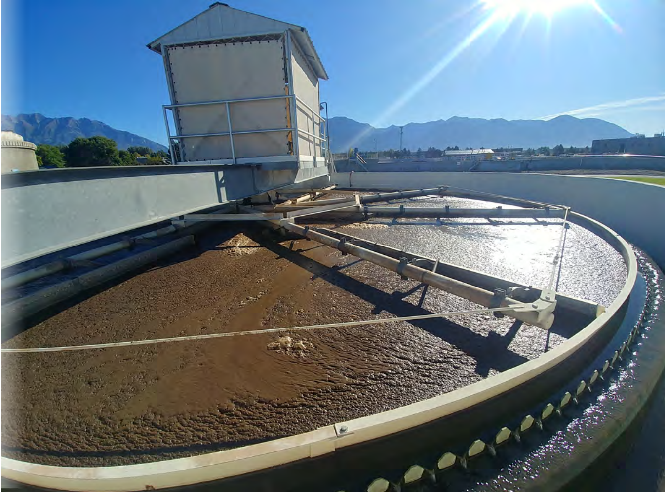
Figure 8: Dissolved Air Flotation (DAF) thickener open to the atmosphere
