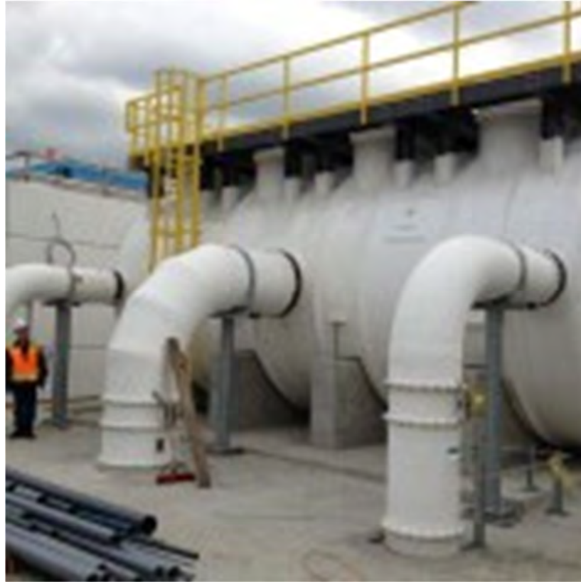
Figure 15: Horizontal Bed Carbon Dry Media System
