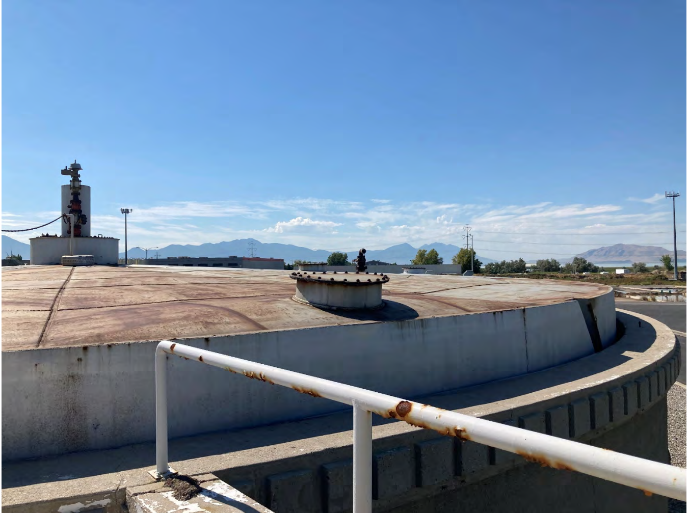
Figure 26 – Floating cover and mixer on mesophilic digester
