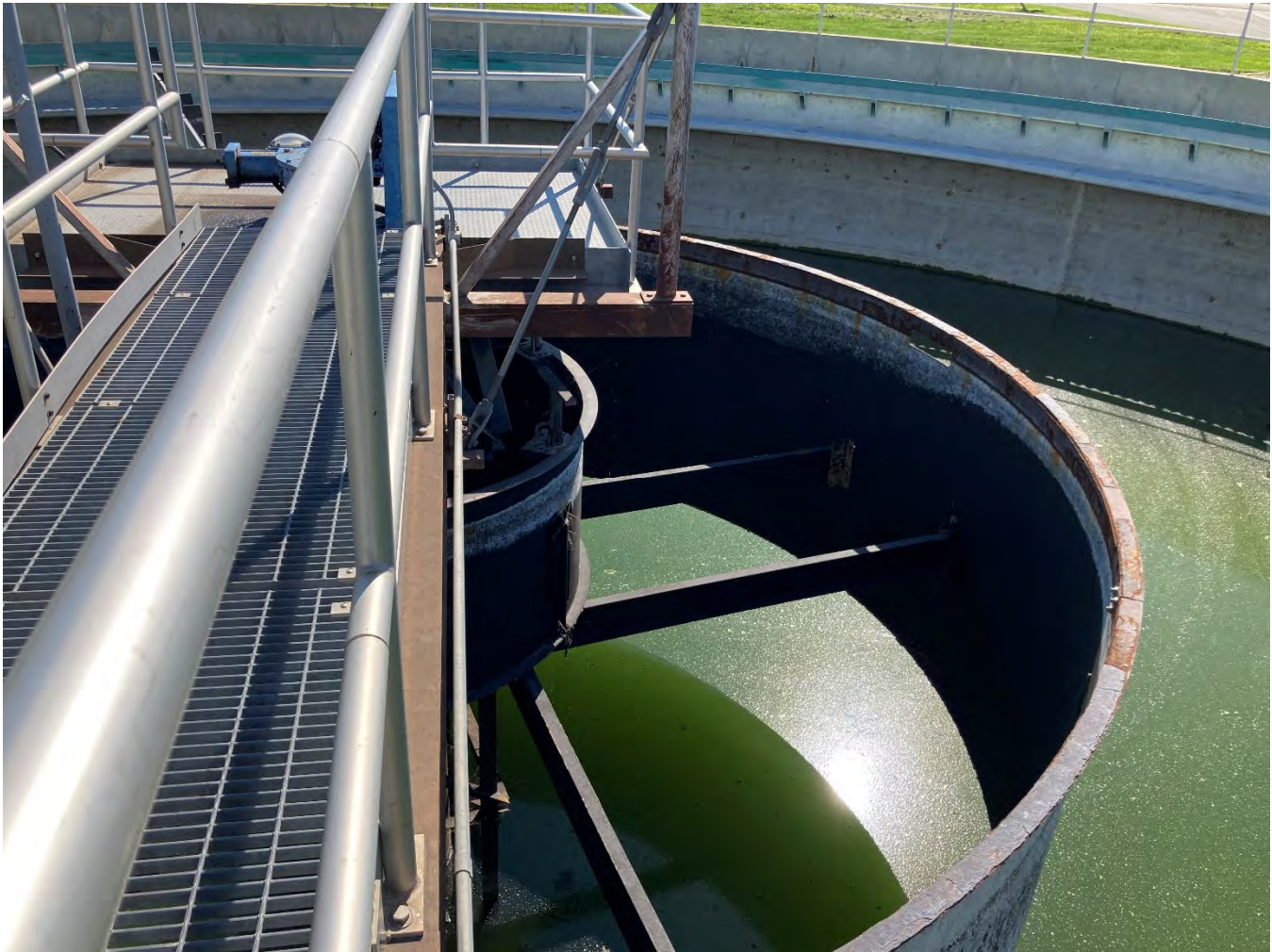
Figure 19 – Clarifier No. 5 Center Well
