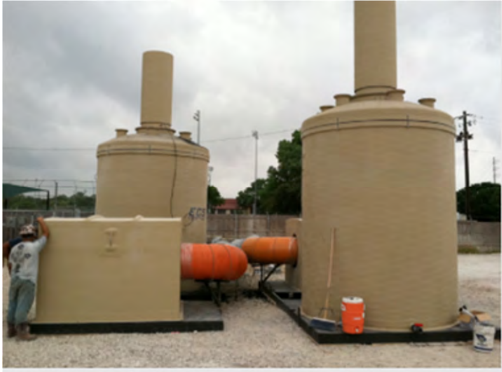
Figure 14: Vertical Bed Carbon Dry Media System
