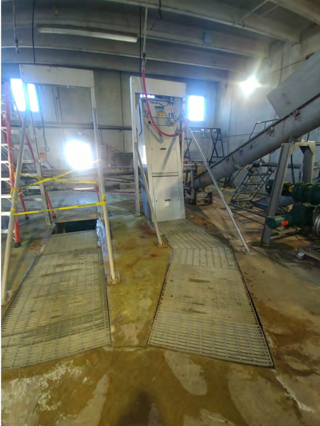
Figure 4: Headworks building with gratings on channels and covered equipment
