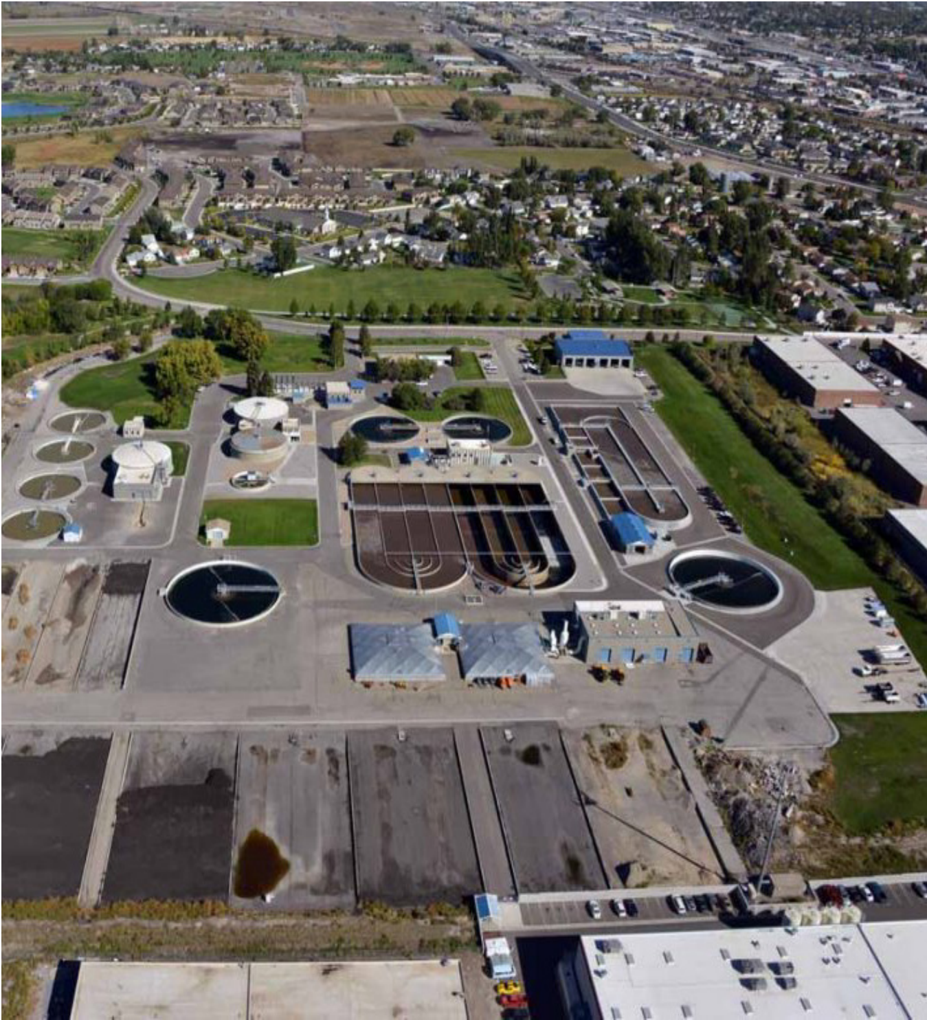
Water Reclamation Plant
