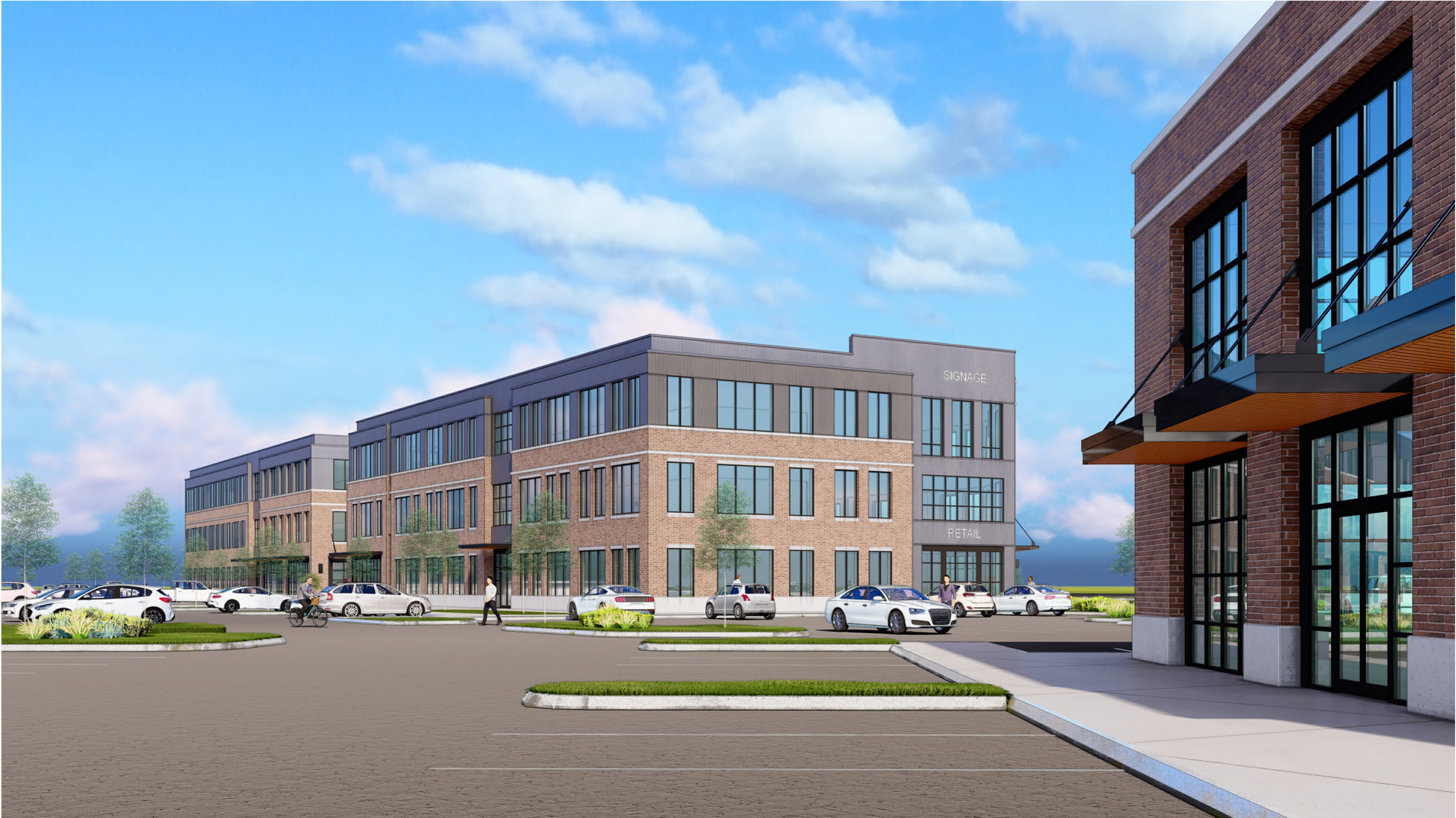
Internal site view to the Northeast
