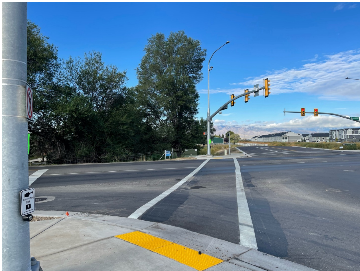
Figure 12: Looking West at Geneva Road / 2000 South
