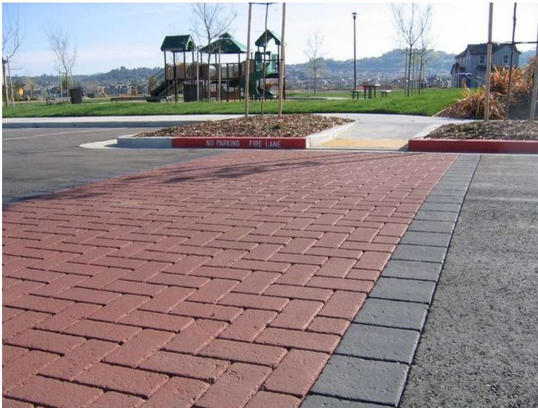
Fig. 9 Stamped and colored asphalt.
