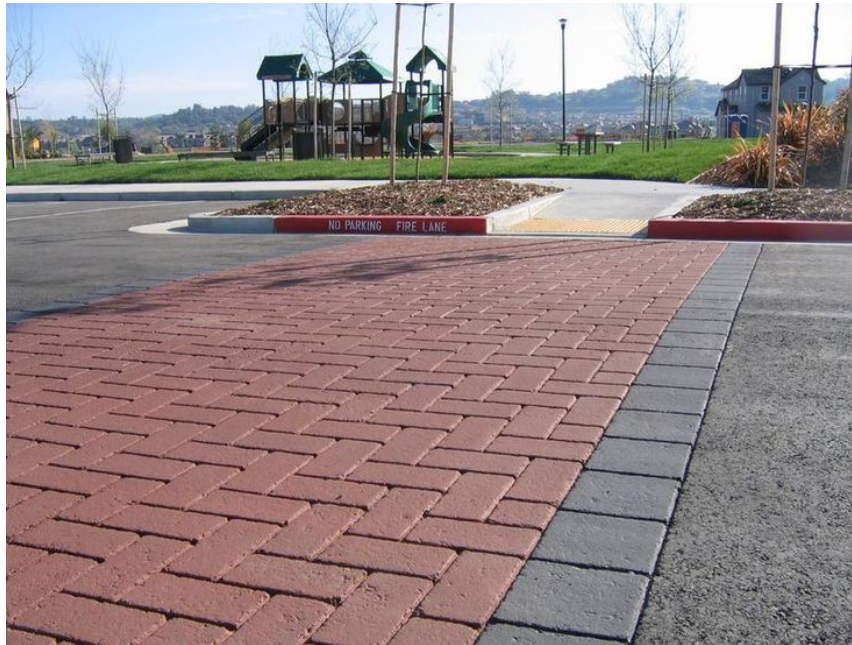
Fig. 9 Stamped and colored asphalt.
