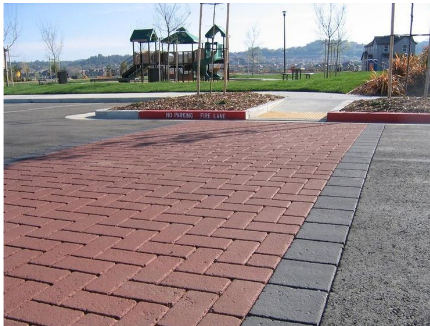
Fig. 9 Stamped and colored asphalt.
