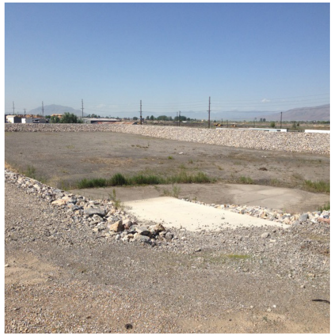
800 North Detention Pond
