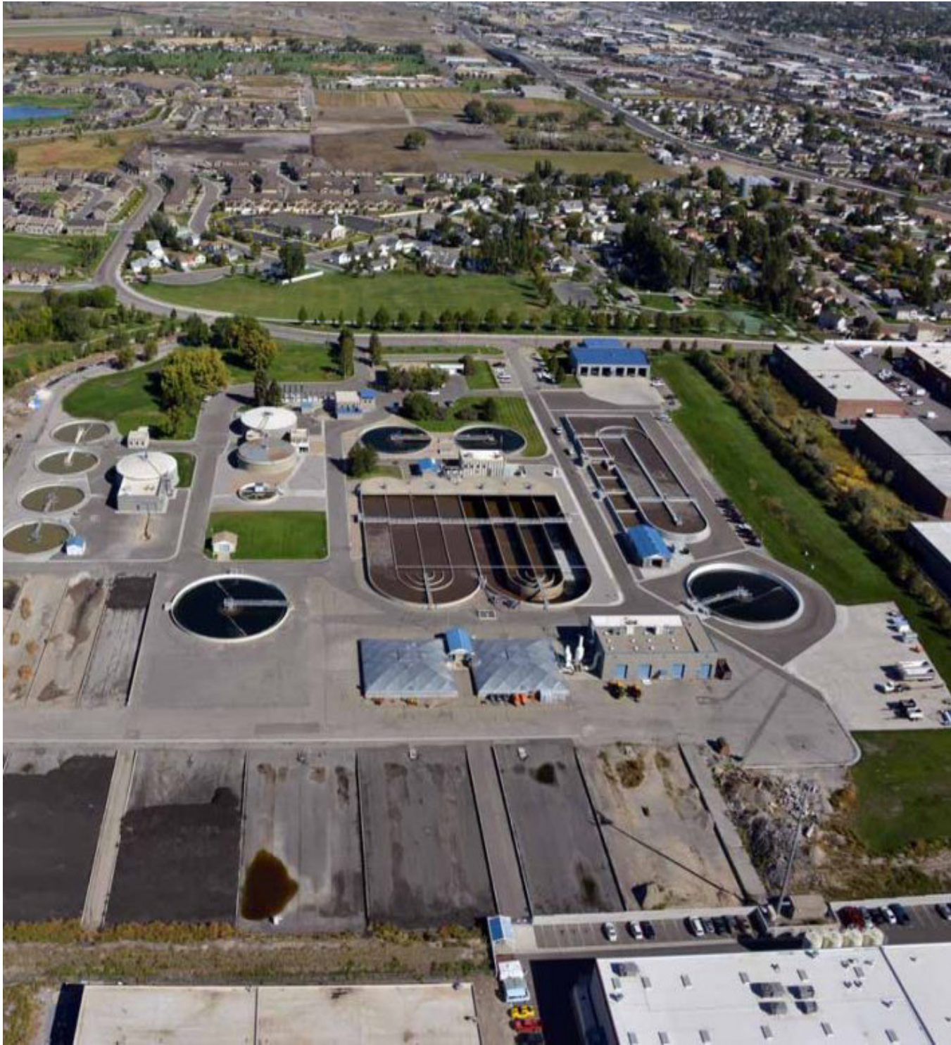
Water Reclamation Plant
